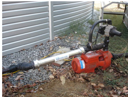
Model T220 Turbu-Flow On Irrigation Pump
